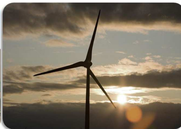
Operation of Wind Turbine Generators
